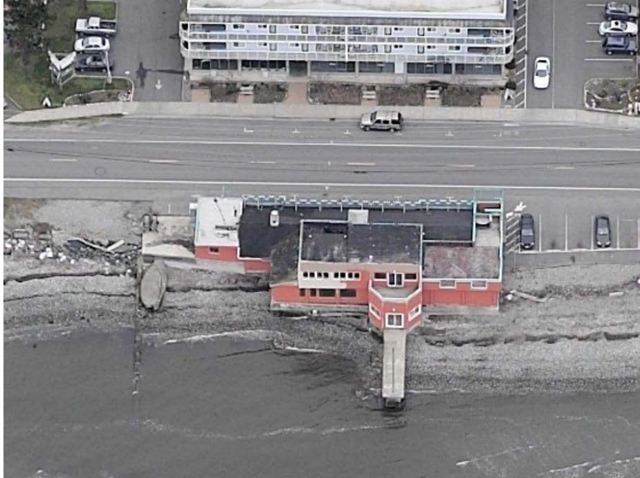
Figure 7: The Birch Bay Bistro restaurant in Whatcom County is a legal nonconforming use and structure.
