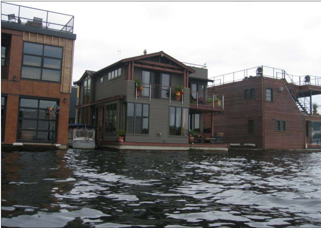
Figure 4: These floating homes in the City of Seattle are connected to city water and sewer and must meet building code requirements. (City of Seattle photo.)
