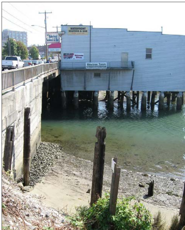
Figure 2: The Waterfront Tavern bar and grill on the Whatcom Waterway in Bellingham is a legal nonconforming use and structure.
