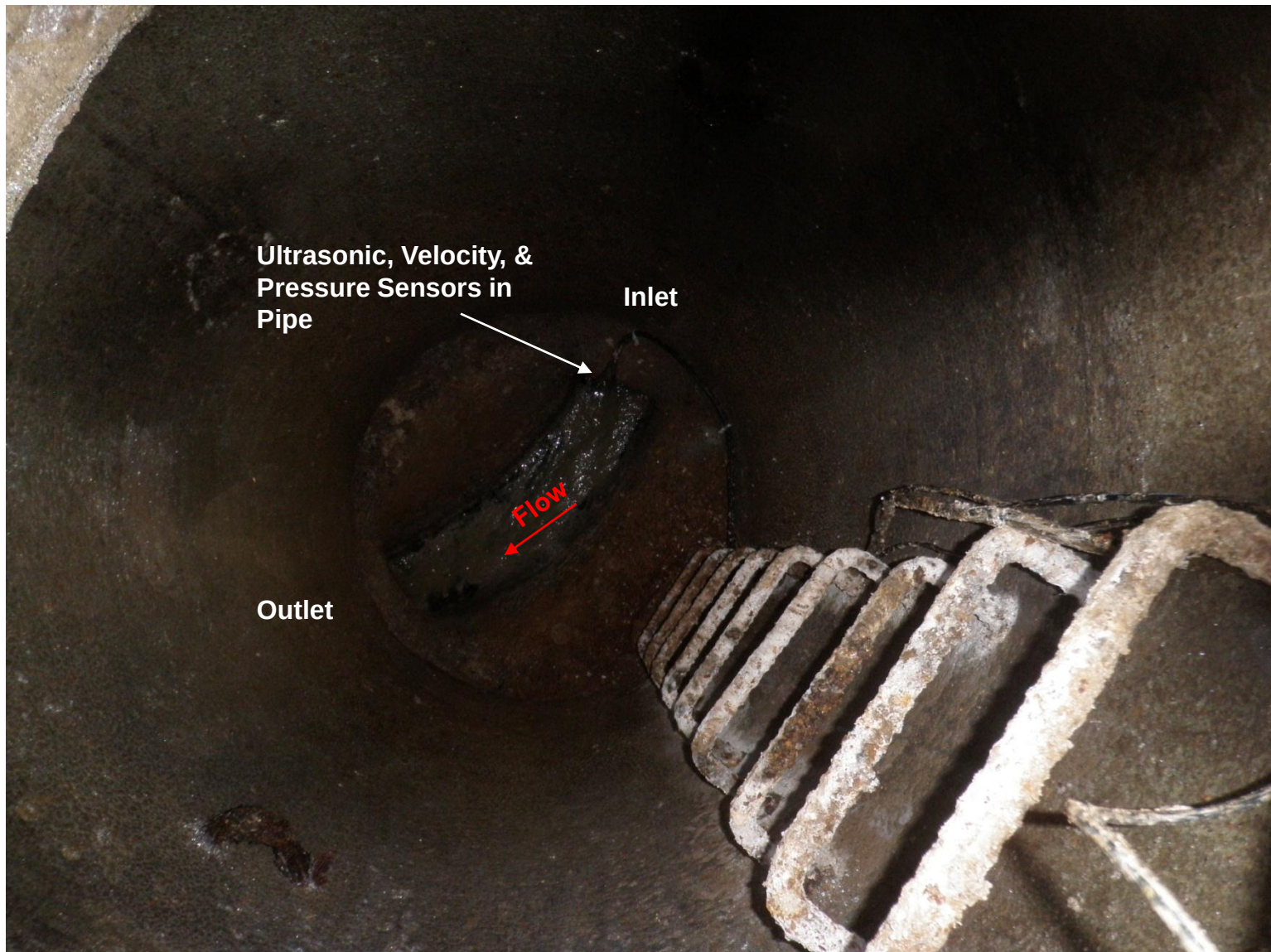
View of site looking north
