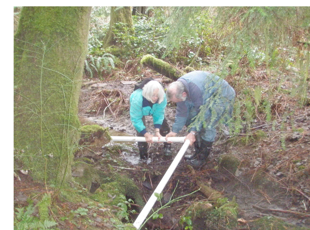
Volunteers installing the gravity-fed piping that brought fresh water through the raceway from upstream.
