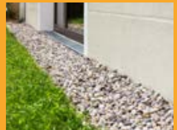
Move any flammable materials like mulch, leaves, pine needles, and firewood piles (anything that can burn) away from exterior walls.
