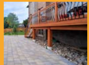
Remove flammable items from underneath decks and porches.
