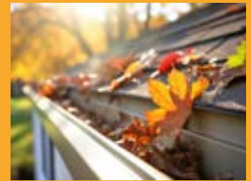
Clean roofs and gutters of dead leaves, debris, and pine needles.
