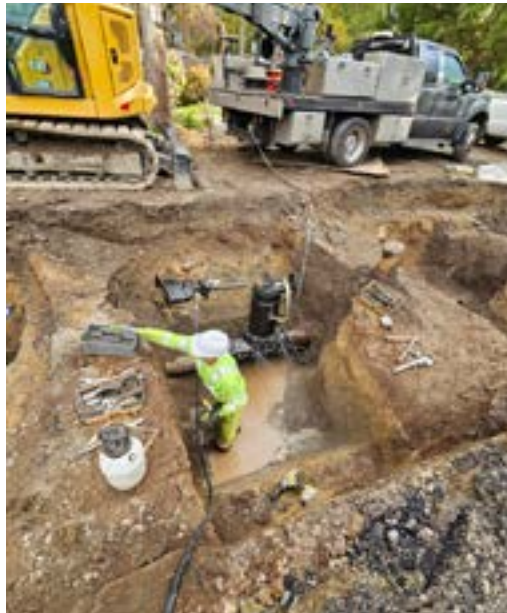
Water upgrades prior to paving in November.
