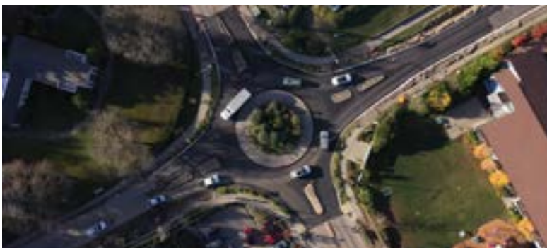
Roundabout at Madison Ave and High School Rd paved in November.
