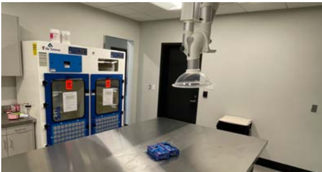
Evidence intake room at Ted Spearman Justice Center.
