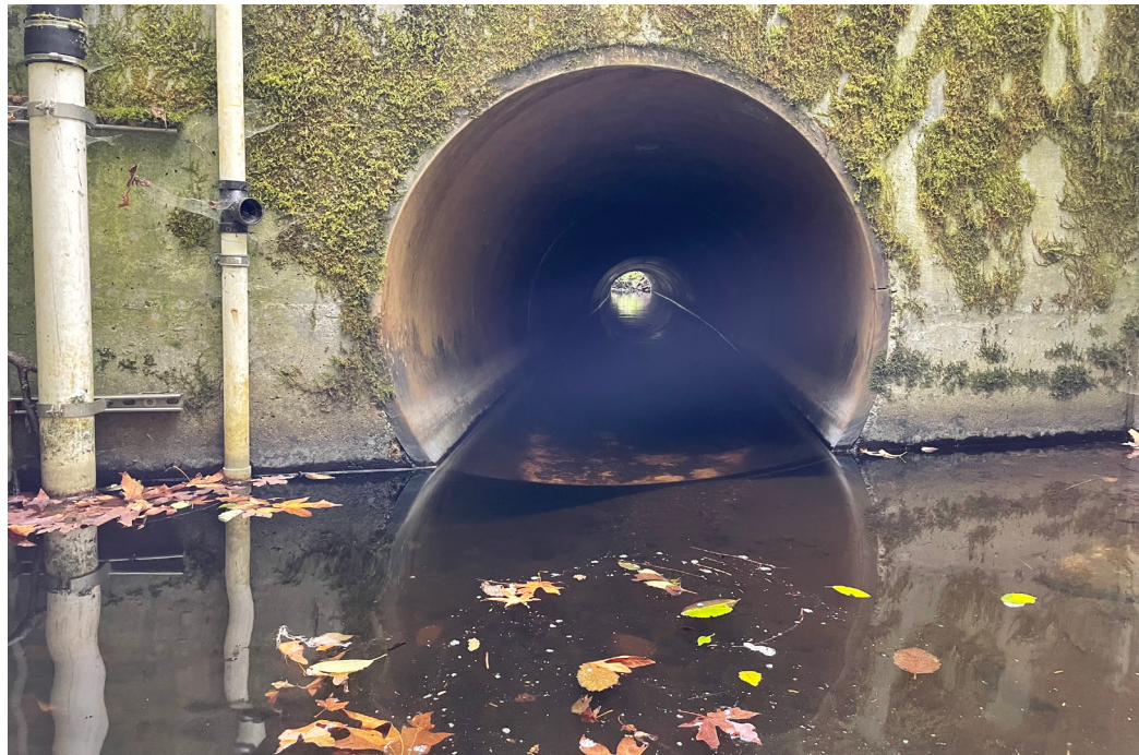
Culvert at Springbrook Creek
