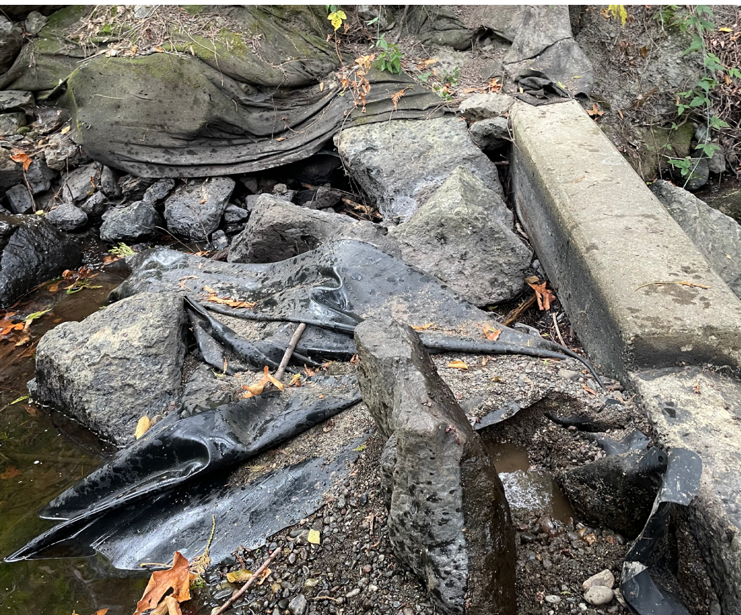
Springbrook Creek Weir during low flow conditions
