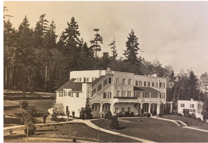
The Moran School's Day Hall, built in 1917 and now known as Messenger House, is located on a bluff southeast of Rolling Bay.
