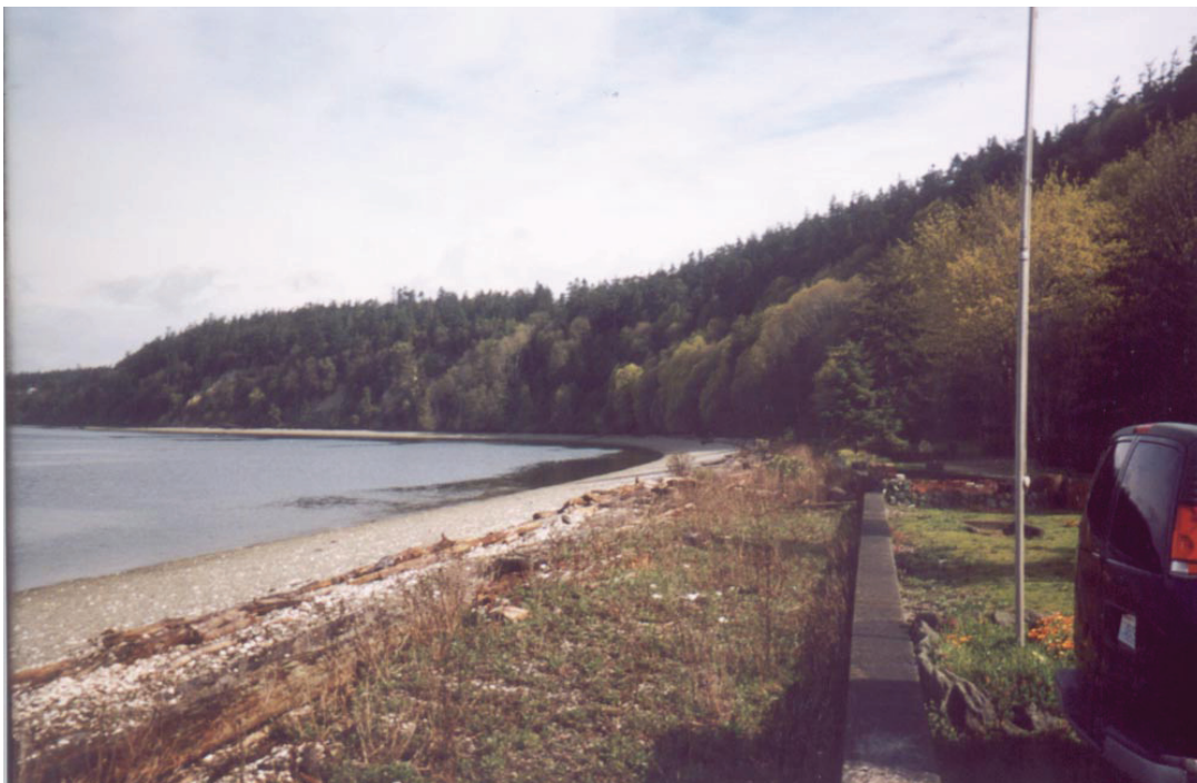
Figure 3. Photograph of Cama Beach where a bulkhead was constructed on an accreting beach. Note upland vegetation (red alder) growing in front of the bulkhead.
